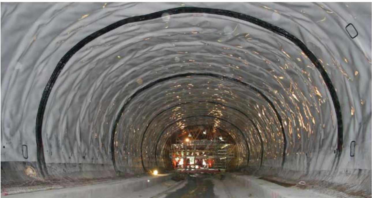
Losenbergtunnel: Absolute Dichtheit für Generationen dank AGRUFLEX. Best water-tightness for generations with the AGRUFLEX tunnel liner.
